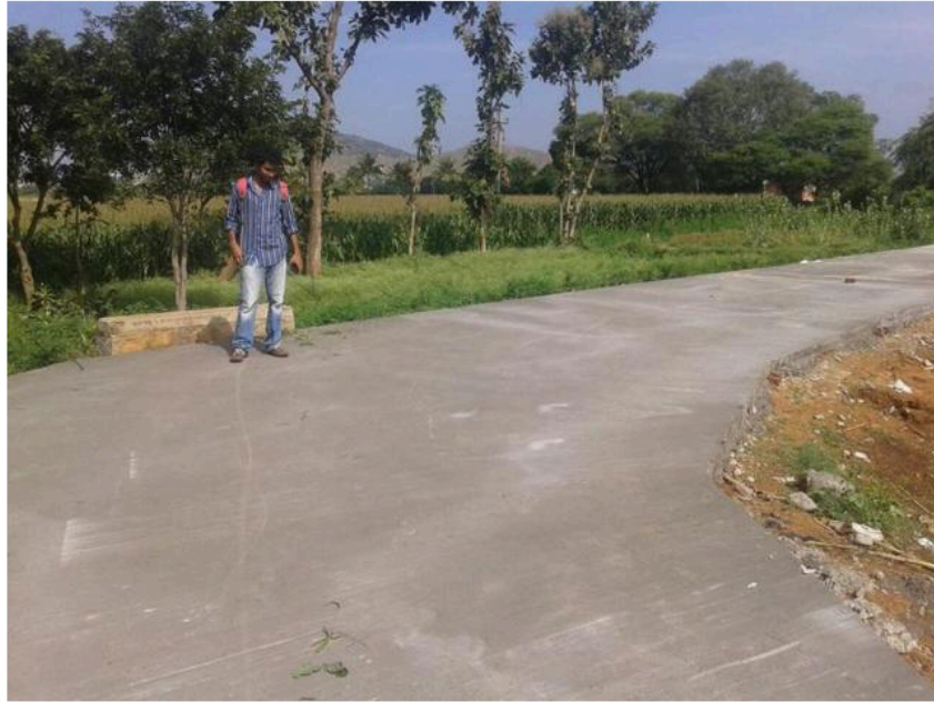
The new self-repairing road that connects Thondebavi village to the highway. (Courtesy UBC)
